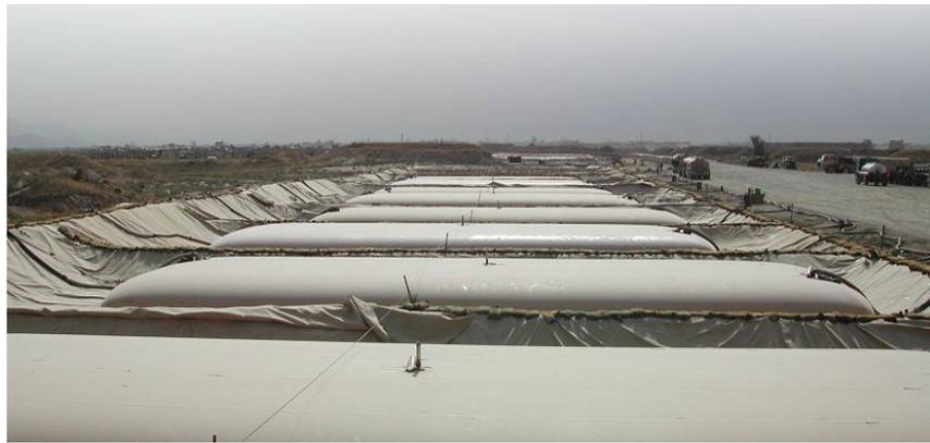
*Once deployed, collapsible storage tanks are simply unrolled into a dike system and filled on site.*
